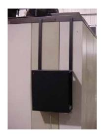
8. Secure the two (2) P/N 216H559 black box hanger brackets to the top rail as shown using the (Wenger P/N X001192) ½" diameter by 1" long, hex washer-head self-drilling screws supplied in the kit with the hanger brackets. These screws have a metal-cutting drill point that is designed to be drilled directly into the ceiling rail of the Wenger VAE sound isolating room using a standard drill driver with a 3/8" hex driver bit without the need to pre-drill pilot holes in the ceiling rail.
